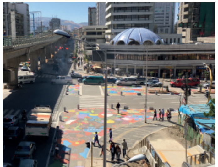
The lanes at LeGare were aligned to make vehicular movements more organized and reduce points of conflict. Reclaimed roadbed space was transformed to provide refuge for pedestrians.*
