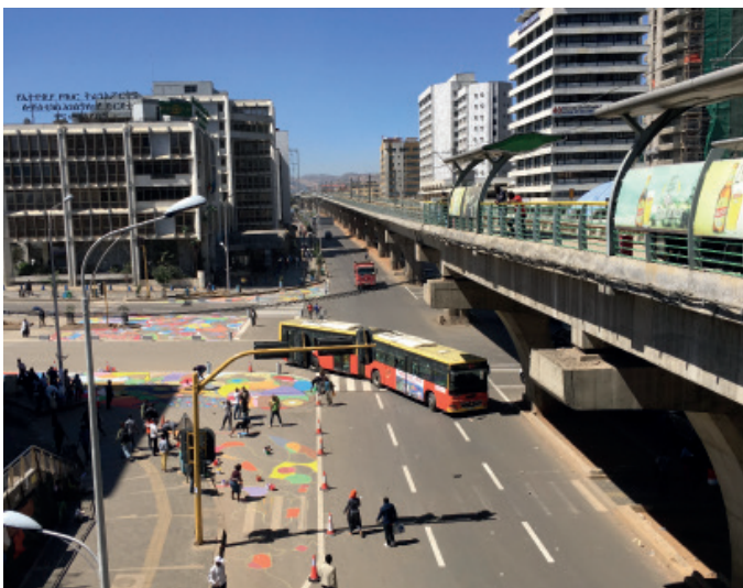
At LeGare, the turning radii was reduced from 16m to less than 7m, still allowing for large buses to turn at safe speeds.*
