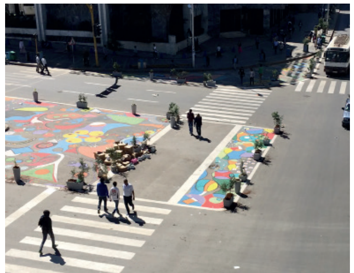
At LeGare, refuge islands have been used to provide safe spaces for pedestrians and reduce crossing distances for all.*
